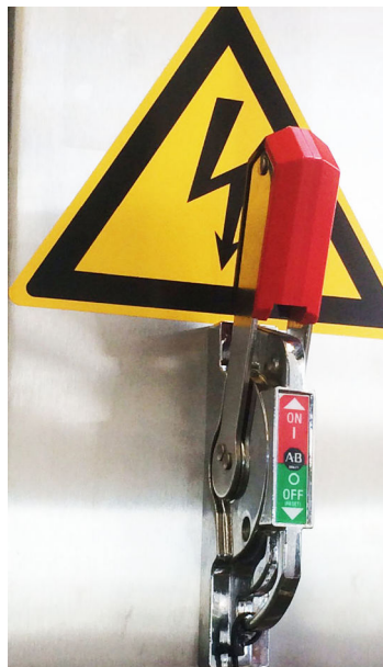
Figure 169: Main switch (example)
